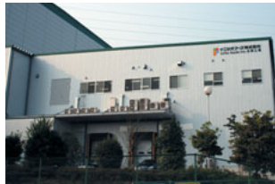
Initio Foods' Shiraoka Plant
