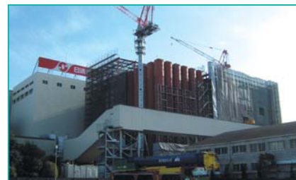
Line expansion construction for the Higashinada Plant
