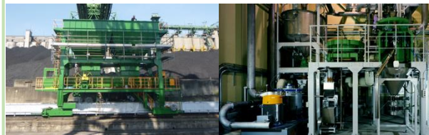
Biomass fuel facility
